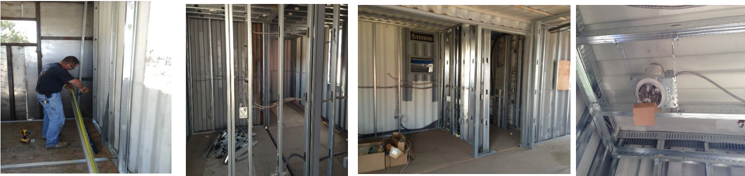
Install Interior Framing as shown
