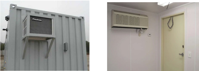
Install heating & cooling systems as shown
